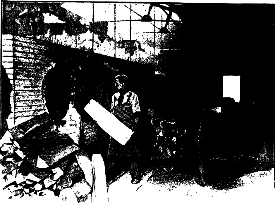
THE CHARCOAL FACTORY: CHARGING THE CYLINDERS.
